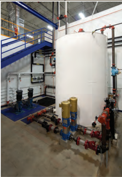
A 4,000-gallon water supply tank provides ample process water to maintain engine temperatures throughout test sequences.
